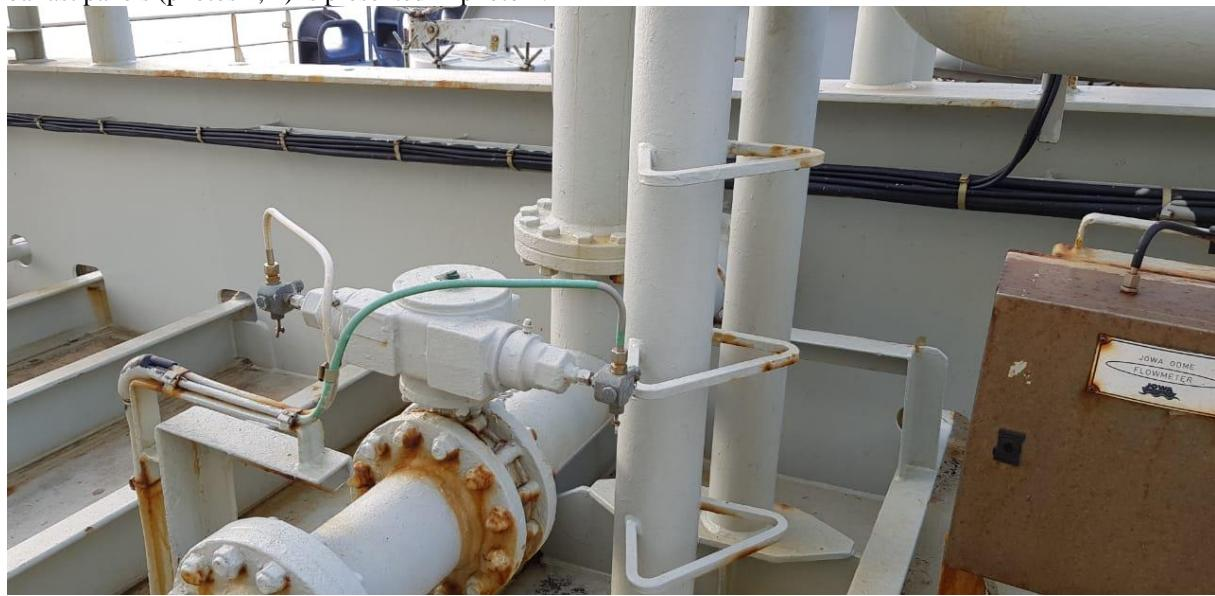
*Photo 4. Electro-hydraulic valve.*
